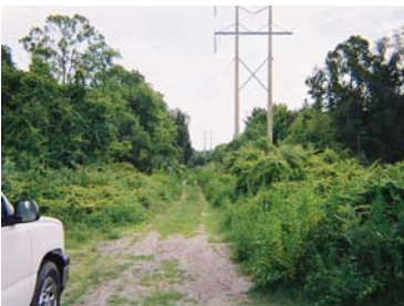
Figure 8: Undeveloped utility corridor looking east.
