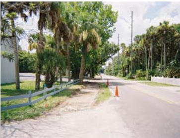
Figure 6: Sidewalk construction on Saxon Dr.
